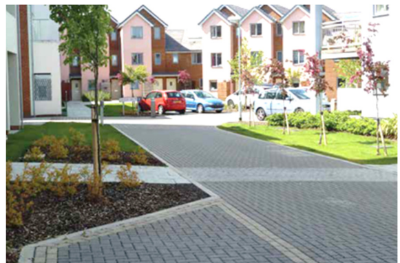
Figure 4-4: Image of Permeable Paving
