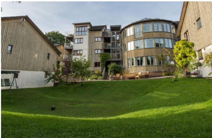
Figure 4-6 An image of a Detention Basin
